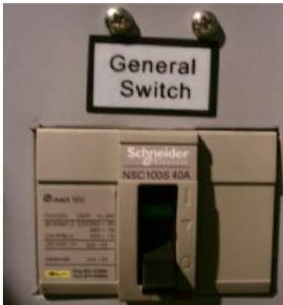
Before running the machine, please turn on the this switch. After the machine is stop, please turn off the this switch
